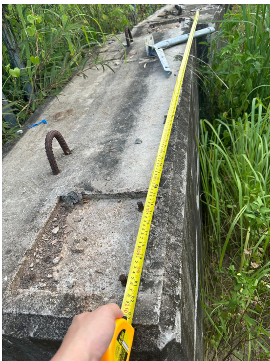
PHOTO 3-5 Site photo for the concrete block type 1 to be removed
